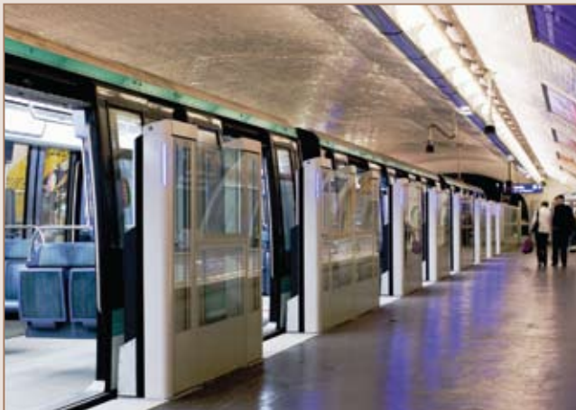
Left: Half-height platform screen doors prevent intrusions – a major source of disruption. Right: Drivers of lines that have been automated can be promoted to the Control Centre.
